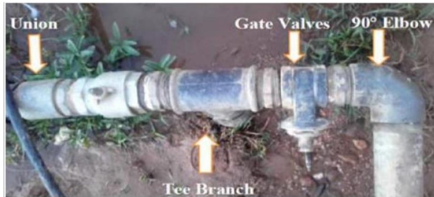
Figure 6. Sample of the minor fittings available in a section of the network available at the Hamelmalo Agricultural College farm. Source: [11].
